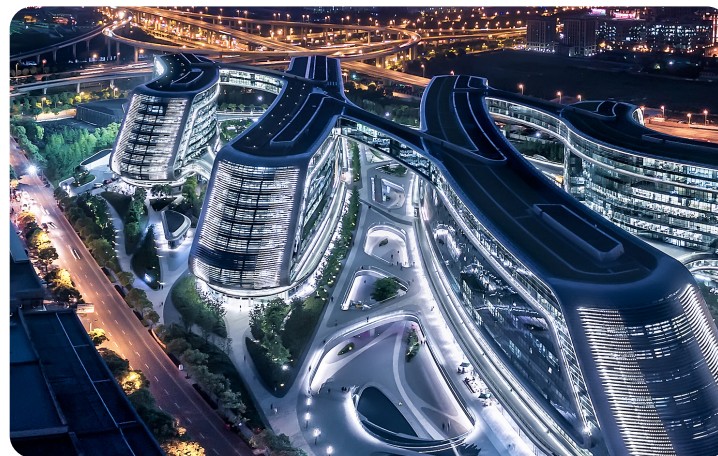
Trip.com Group's headquarters, SKYBRIDGE HQ, has earned the "Leadership in Energy and Environmental Design" and a LEED Gold Certification.
